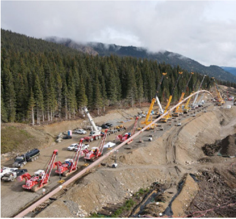
Figure 5 - Pullback execution
