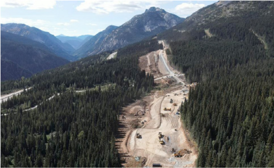
Figure 3 - Preparation of Launching Platform and drilling Pad
