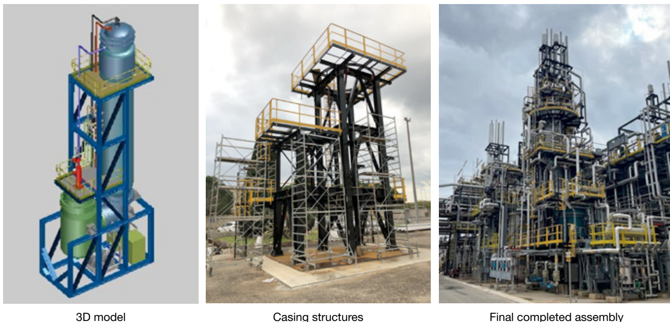
Figure 6 – Taranto plant from 3D model to operational in refinery
