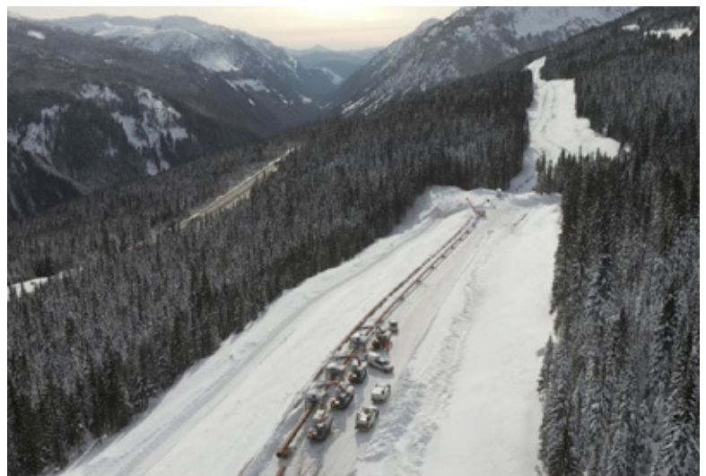
Figure 4 - Secondary strings pre-fabrication
