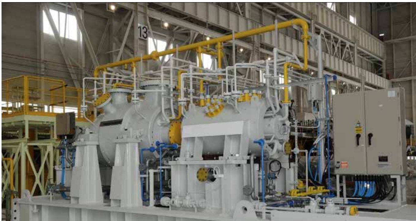
Gearbox and compressor
