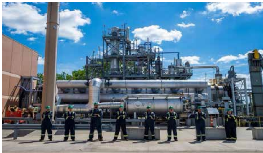
Alterra Industrial facility in Akron-OH
