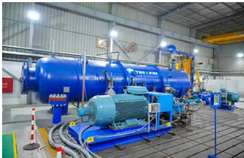
Trillium's new pump manufacturing facilities in Al Jubail – test center
