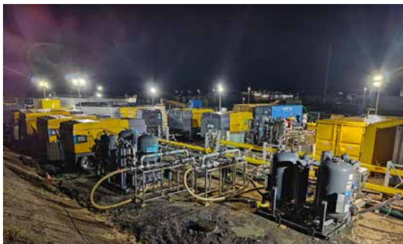
Equipment layout at Ostsee Anbindungsleitung (OAL) pipeline's pre-comm site
