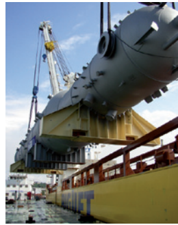
Lifting operation of a Amine Absorber (dimensioni: cms 3959 x 806 x 800 – up to 398 Tons / Unit);
