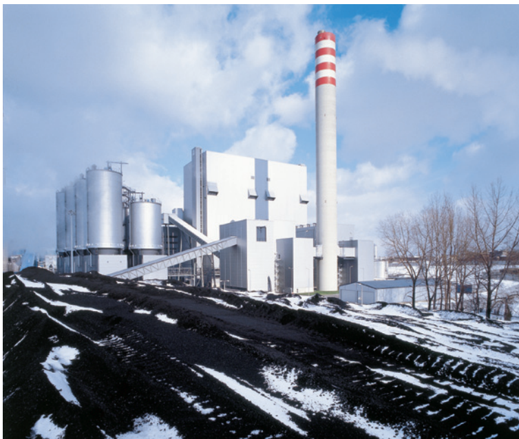
Coal Power Plant designed and built by Foster Wheeler for Elcho at Chorzow, Poland
