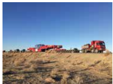
Modernization of Talimarjan and Tashkent thermal power plants
