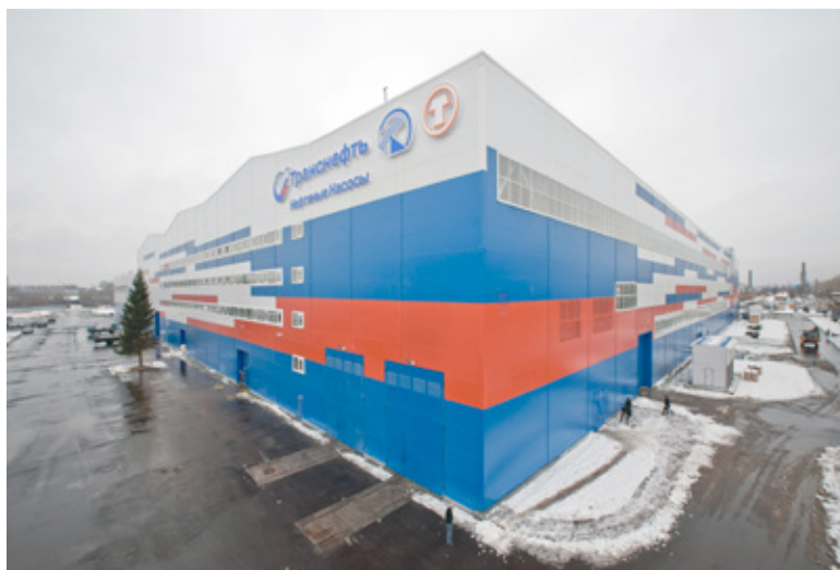
Transneft Oil Pumps facilities in Chelyabinsk: external view
