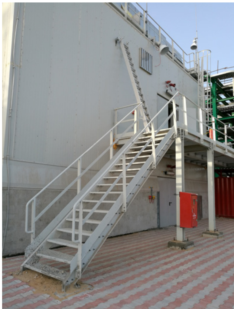
Fig. 2 – A view of Electrical Power Module Building
