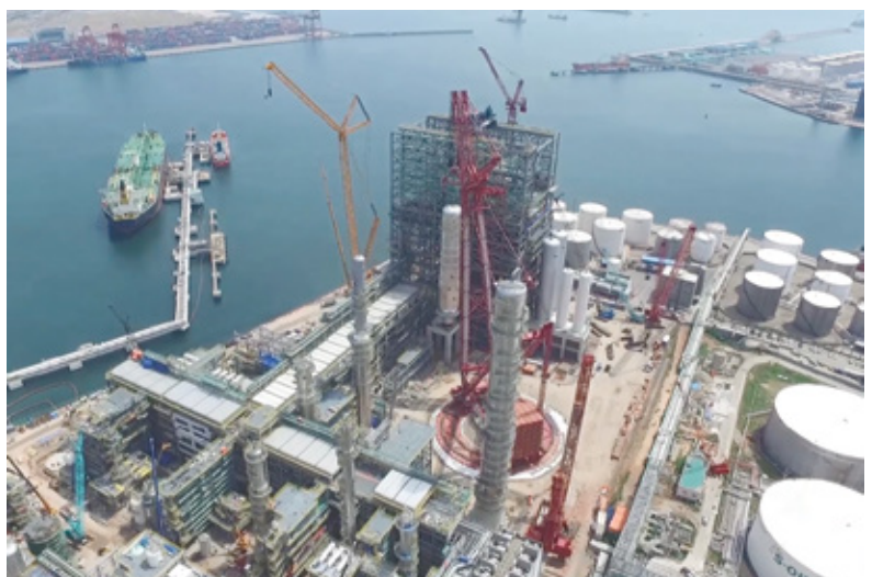
Ring crane installation of-the final column
