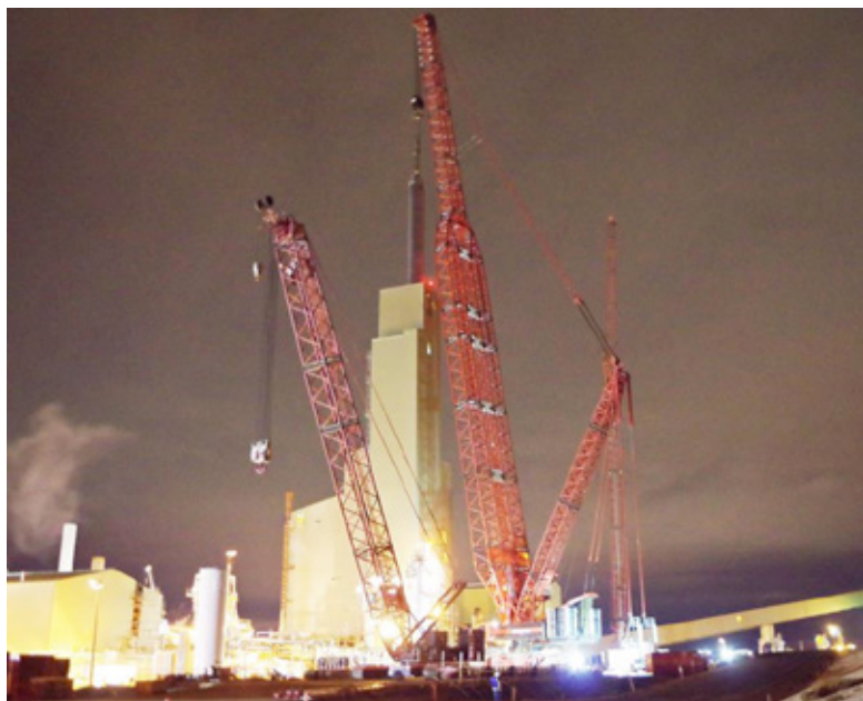
Fertilizer vessel installation
