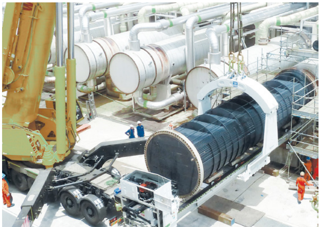
Fig. 3 – MEF express: aerial tube bundle puller
