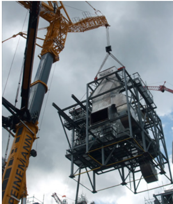
Fig. 9 - Layout and pictures of the lifting of two modules, including the biggest one (~100 tons)
