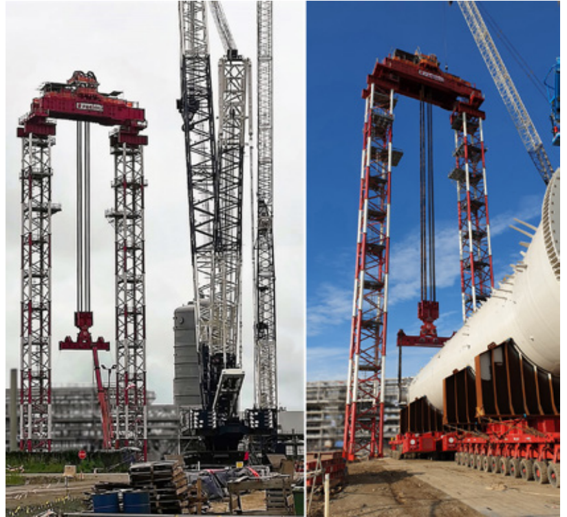
Picture 7 - Fagioli tower lift and strand jacking system
