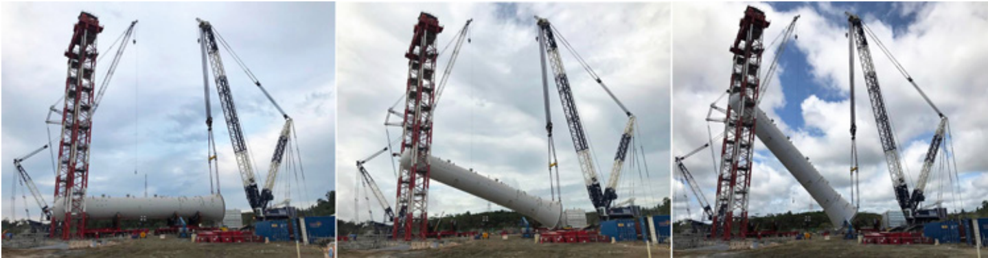
Picture 11 - Lifting operation
