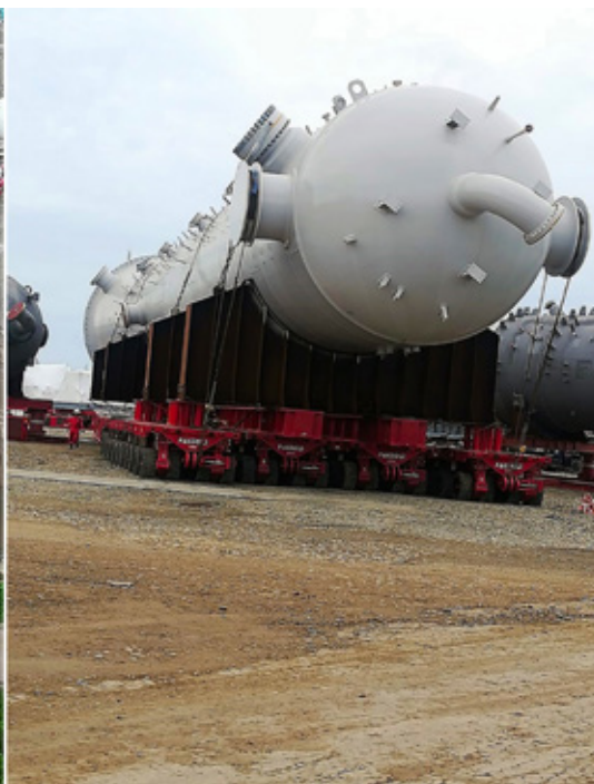
Picture 8 - Detail of the Acid Gas Absorber before the lifting operation
