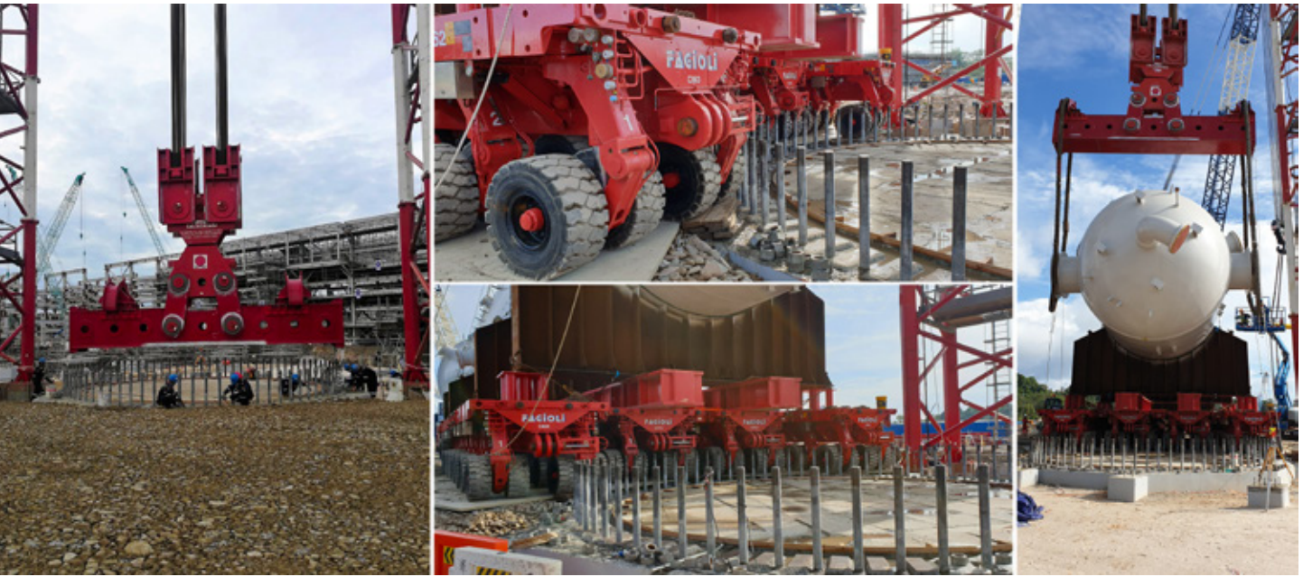
Picture 9 - Connecting the Acid Gas Absorber to Fagioli tower lift system
