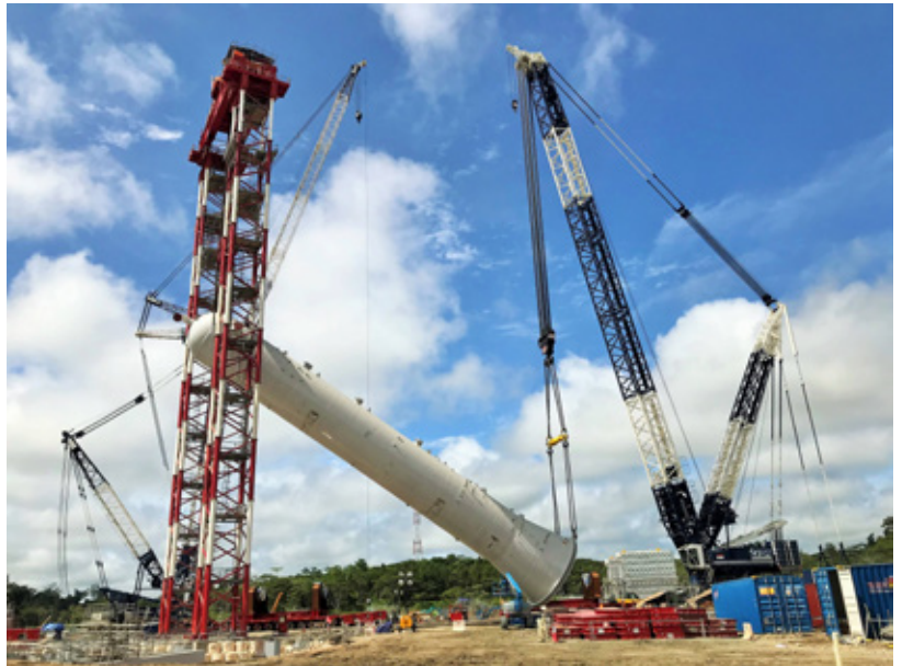
Picture 12 - Lifting operation (Detail)
