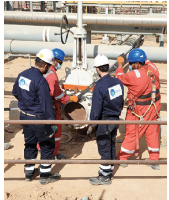
Fig.2 - Bolt Tightening with Manual Wrench
