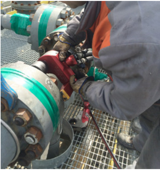
Fig. 3 – Bolt Torquing with Hydraulic Tools
