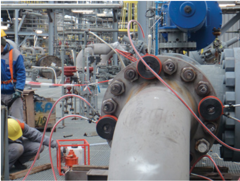
Fig. 1 – Bolt Tensioning
