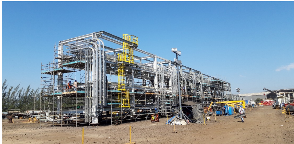
Figure 38 Module under fabrication
