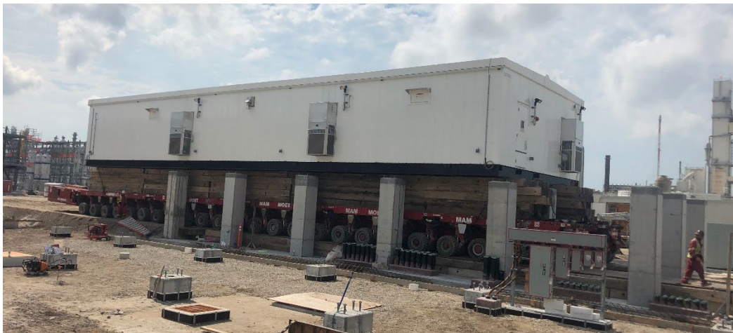
Figure 44 Modularized building installation with SPMT
