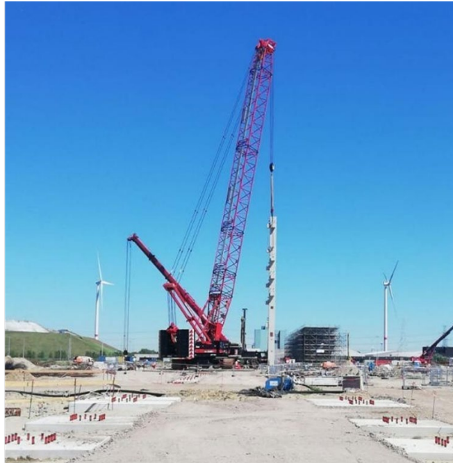
Figure 53 Erection of column with a full precast approach
