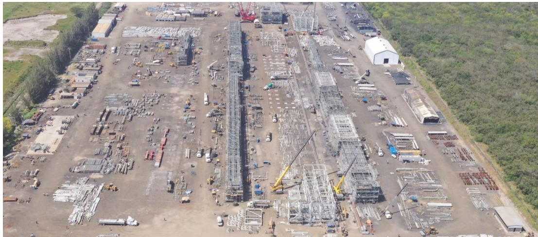
Figure 40 Aerial view of a fabrication Yard
