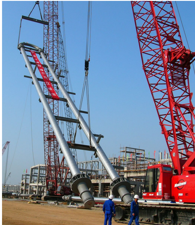
Figure 29 Lifting operation for Loop Reactor
