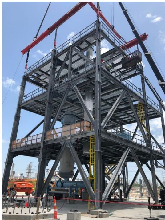
Figure 49 Completion of lifting operations for a pancake's floor
