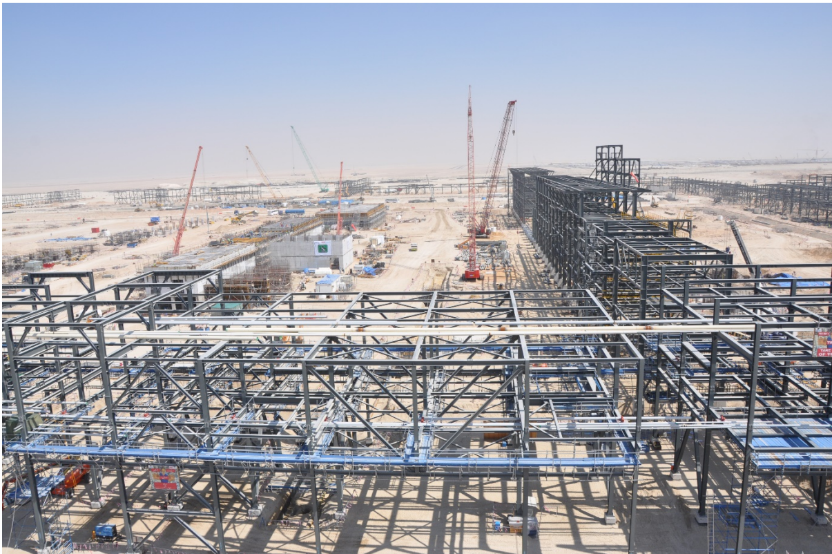
Figure 33 On-going Construction Works
