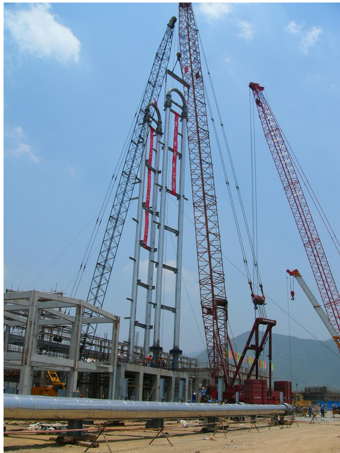
Figure 30 Positioning of Loop Reactor
