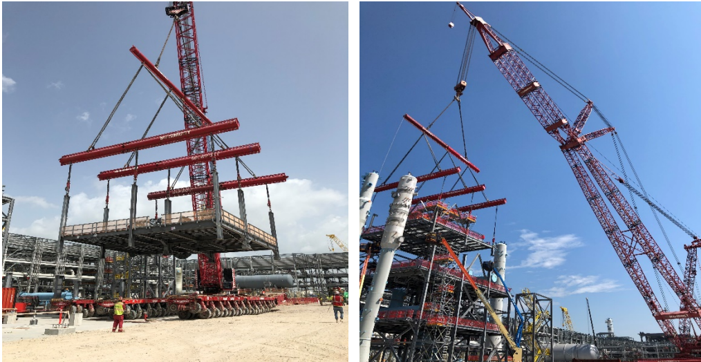
Figure 48 Lifting of a pancake floor
