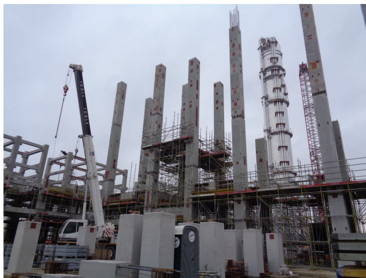
Figure 55 Erection of structure with a partial precast approach
