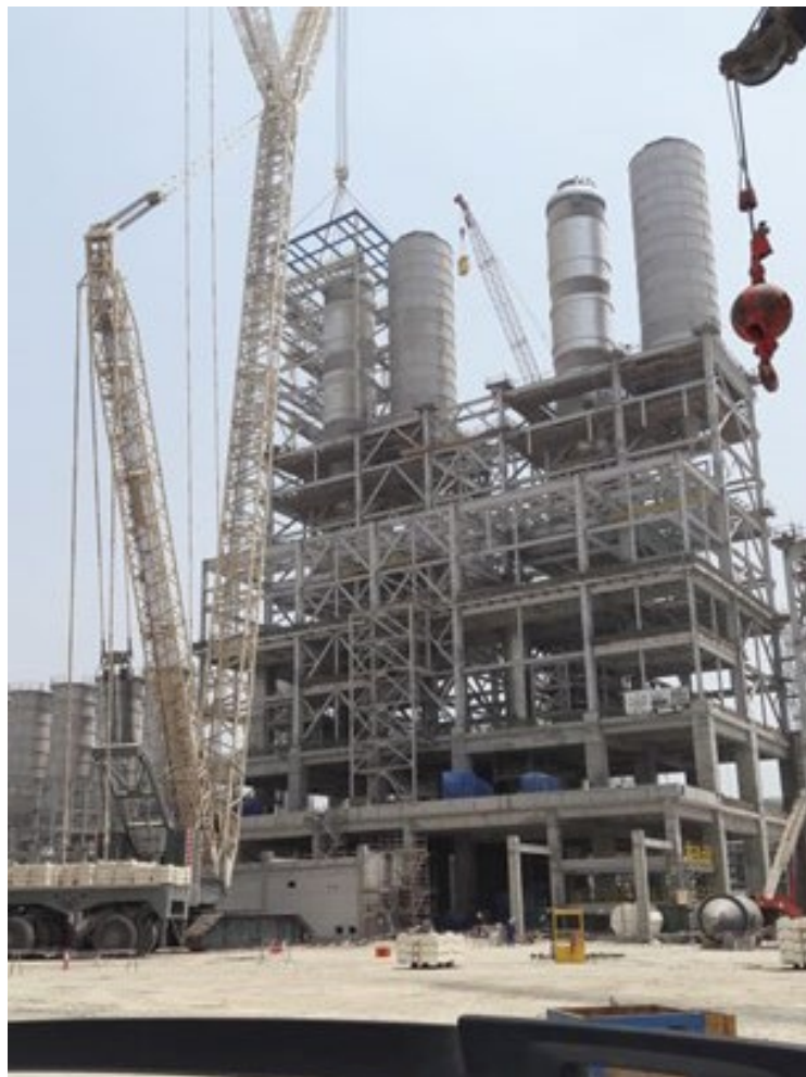
Figure 31 Example of pre-assembled structure installation
