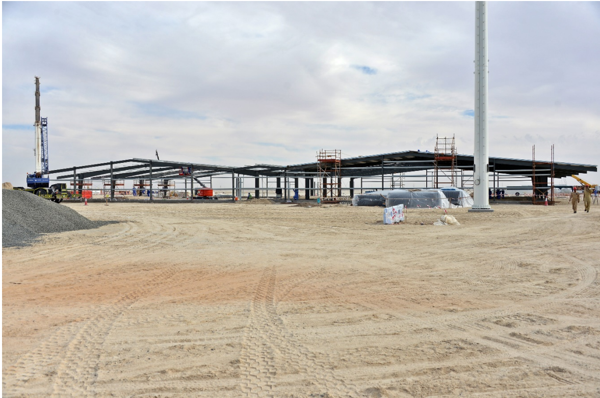
Figure 74 Installation of the Subcontractor's Warehouse workshop, according to Mobilization schedule
