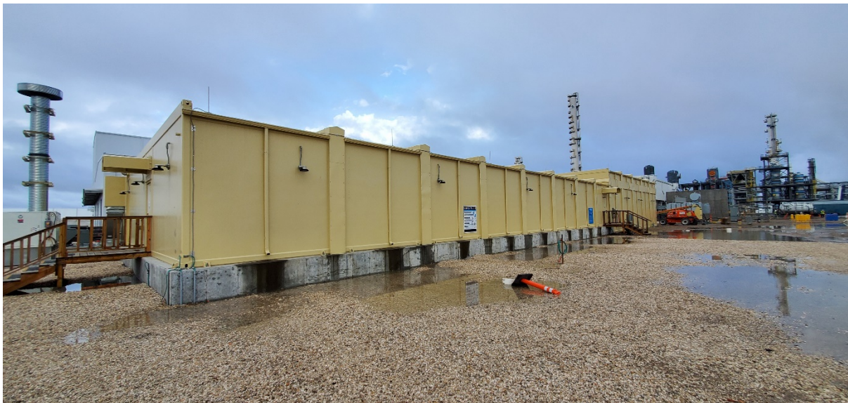
Figure 43 Example of Modularized Control Room
