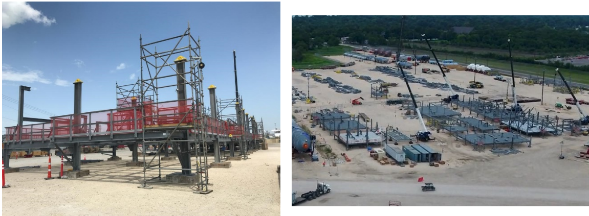
Figure 46 Floor under preassembly
