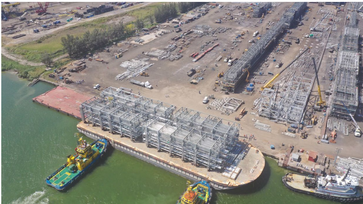
Figure 41 Modules loaded and secured for transportation from Yard to Site
