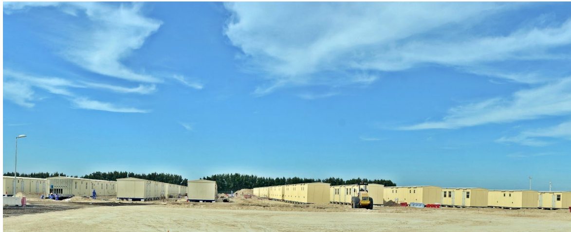
Figure 63 On-going installation of an accommodation camp
